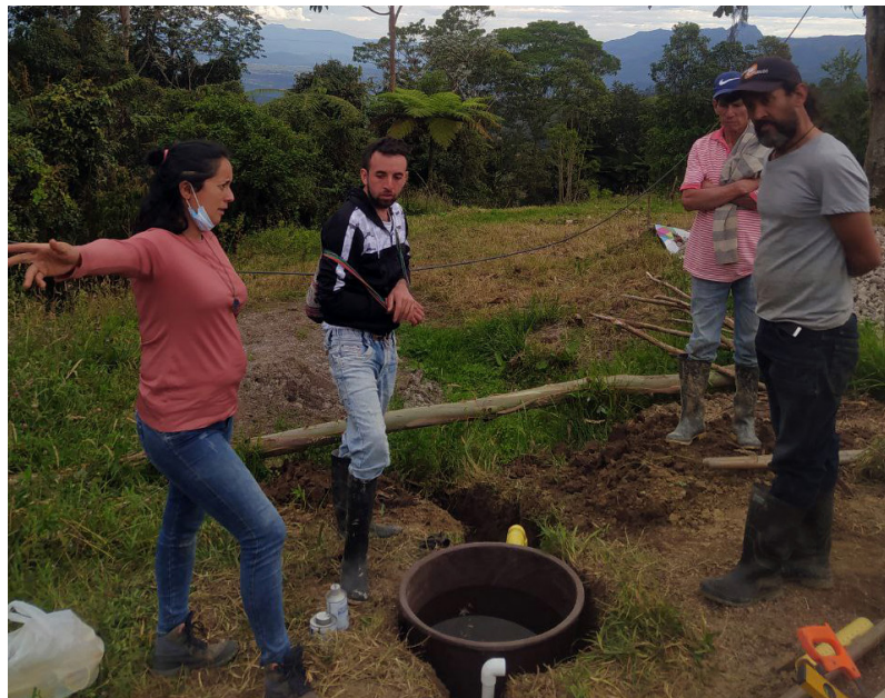
Theoretical-practical workshops and construction of the greywater treatment system version 2.0.
