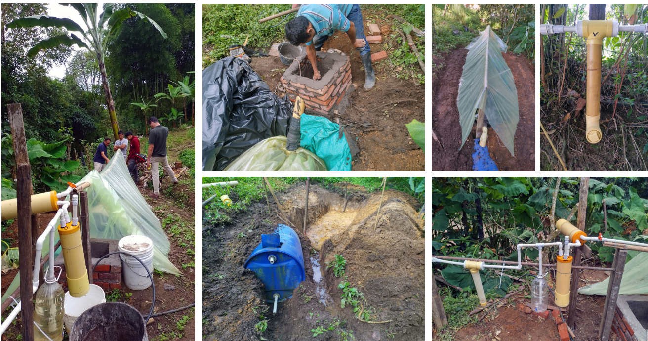
Design, experiments and construction of the tubular biodigester version 1.0.
